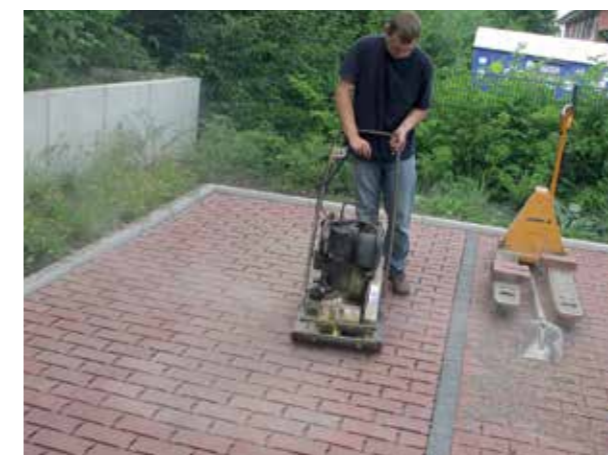
Fig. 5-15: Vibration of the previously swept clinker paver surface with a light vibrating plate
