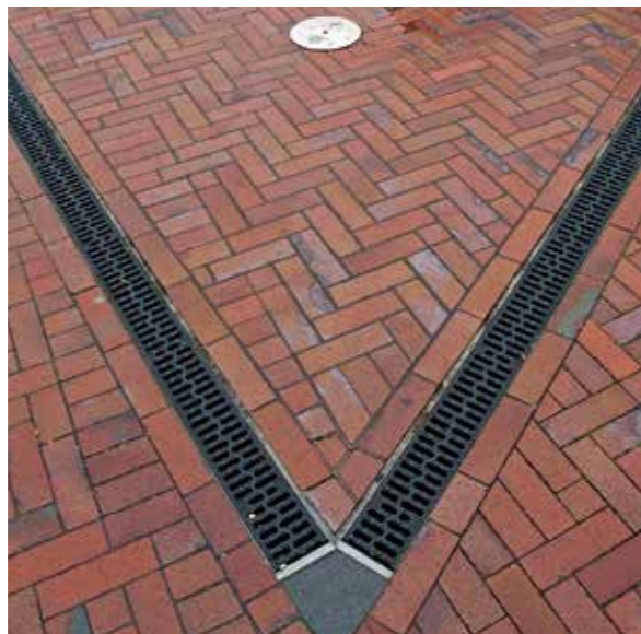
Joint detail – drainage gutter, Barsinghausen, Germany
