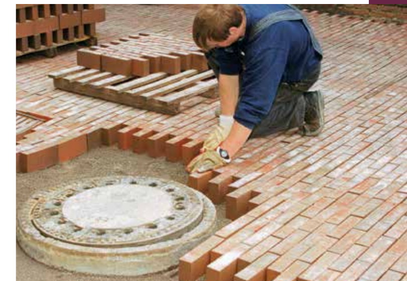
Fitting clinker pavers around manhole covers and drains (installations)
