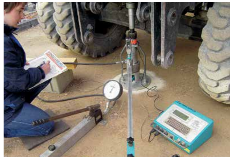
Static plate load test to determine the deformability and load-bearing capacity of the soil
