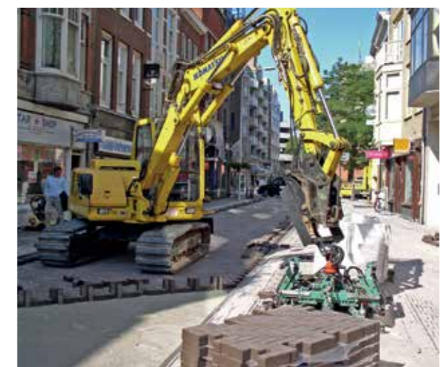
Machine laying of clinker pavers, Den Haag, the Netherlands
