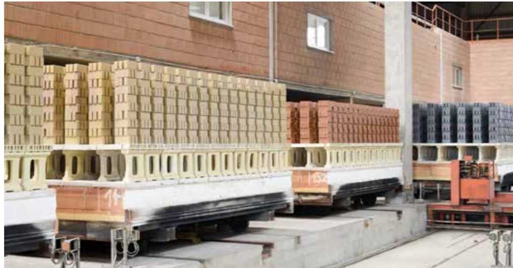
Tunnel kiln car setting with clinker pavers
