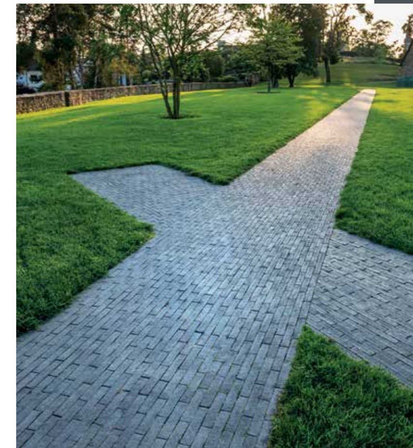
Park way with clinker pavers, laid in a stretcher bond in the walking direction, Lorsch Abbey
