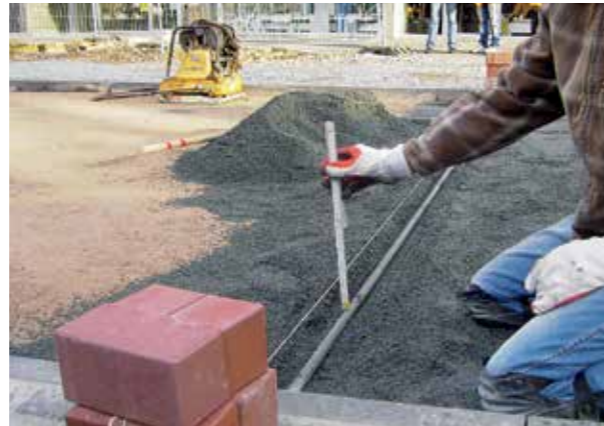
Fig. 5-9: Screeding of the bed surface using previously aligned metal rails
