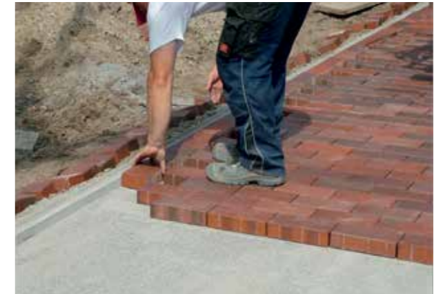
Fig. 5-11: Laying of clinker pavers by hand
