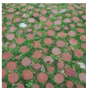
Paving joint – bound with jointing mortar and open to the environment as a greened joint
