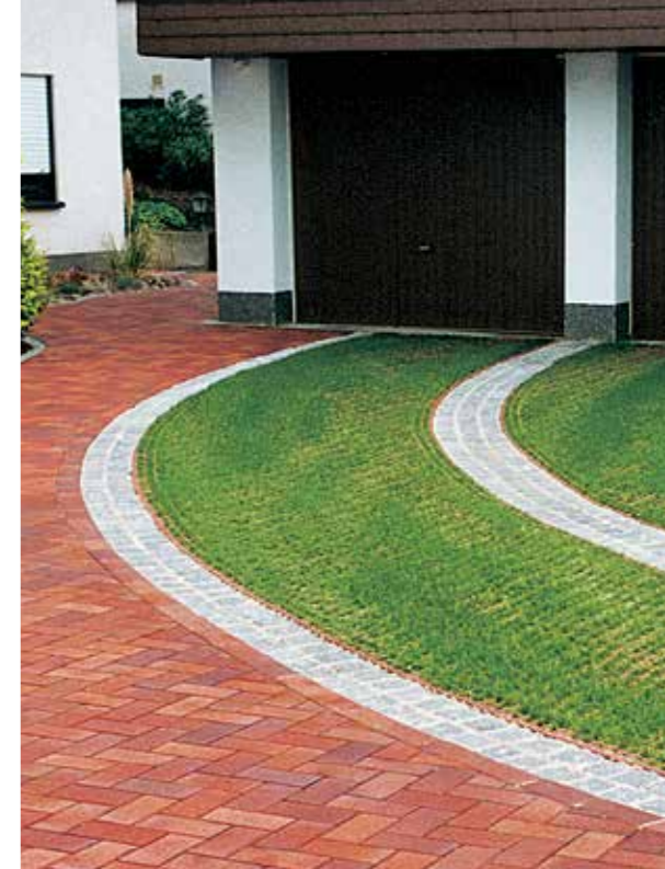
Greened surfaces with perforated lawn clinker pavers
