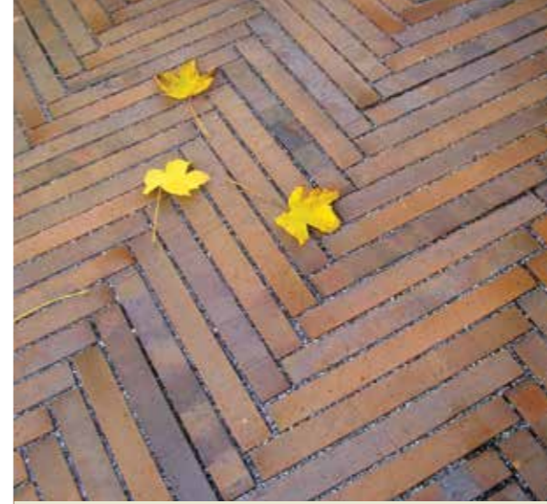
Clinker pavers in a long rectangular shape laid in herringbone bond
